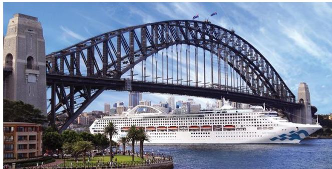
The clearance for shipping under the Harbour Bridge is 45 metres.
